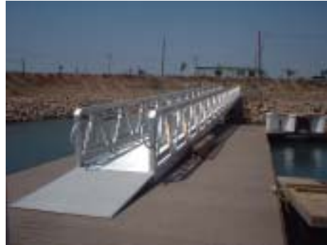
2) Globalgrid Decking as Gangway and Transition Plate
