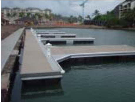
1) Globalgrid Decking as Utility Cover, Knee Bracket and Walkway
