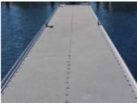
5) Globalgrid Decking as Finger Walkways
