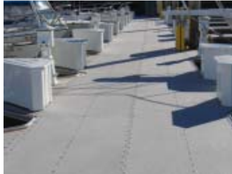
6) Globalgrid Decking as Main Walkways
